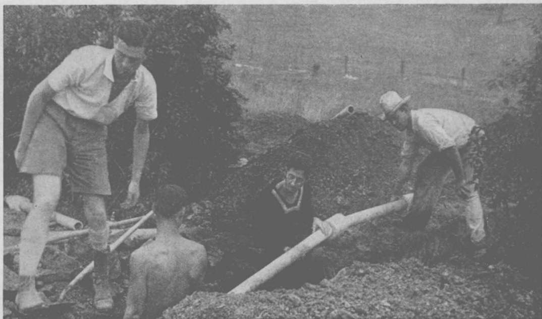
Laying a water system for Penn-Craft Community
