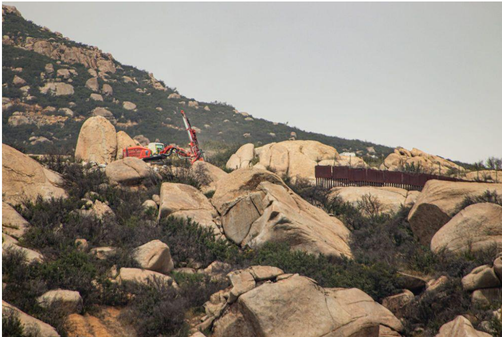
March 2026 construction of the border wall (photo: Pedro Rios)
