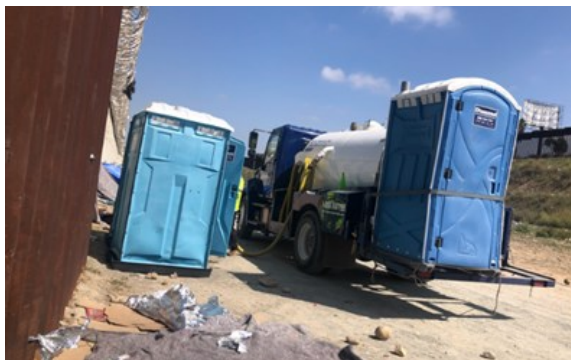
Two portable restrooms between the two 30-ft border walls at Whiskey 8 in San Ysidro, CA
