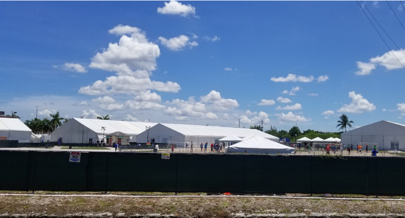
Homestead Temporary Shelter for Unaccompanied Children, 2019. Photographer: Guadalupe de la Cruz.
