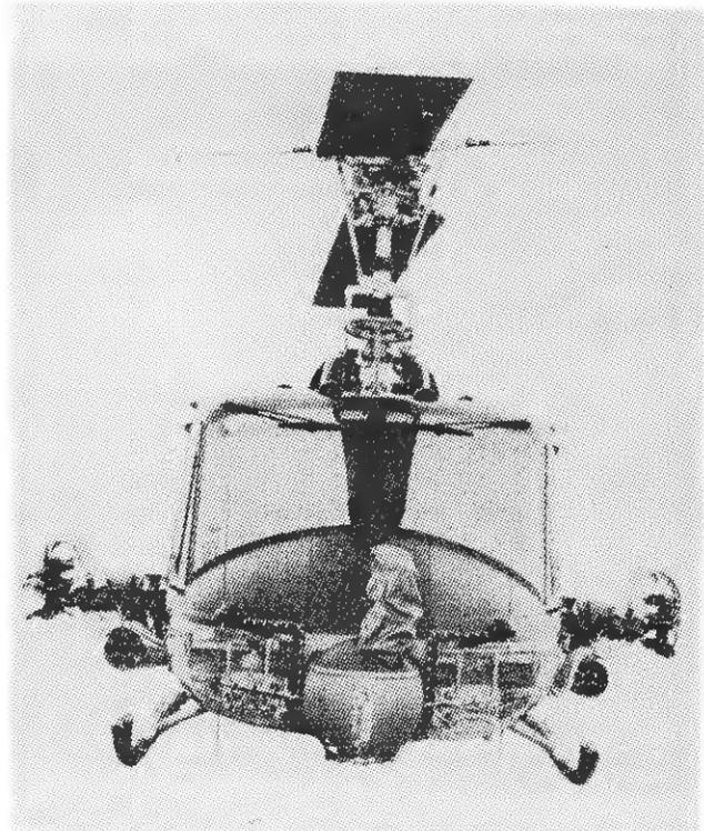
Bell UH-1B with M-5 40mm grenade launcher in nose turret, 2 M-159 2.75" rocket pods, and quad .30 cal. machine guns.
